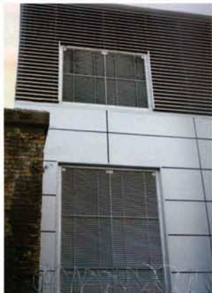
Left: HOSDB approved security louvers, installed at Hoxton, north London; right, Sentinel UltraSecure single door with multi-point emergency panic bar exit system, as installed at Overton in Hampshire
