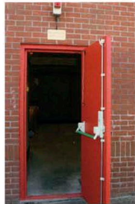
Left: HOSDB approved security louvers, installed at Hoxton, north London; right, Sentinel UltraSecure single door with multi-point emergency panic bar exit system, as installed at Overton in Hampshire
